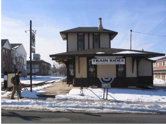
Figure 3.4 — The station for the scenic railway in Gettysburg is an example of Americana found in the small boroughs throughout Adams County.
