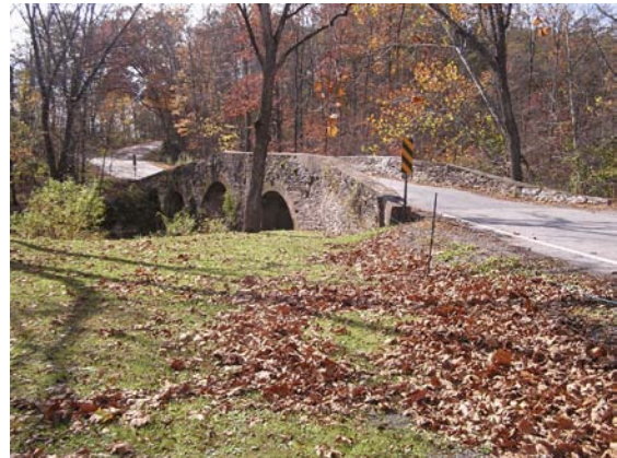
Figure 4 Fig. 2.1 — Historic Pondtown Mill Bridge (see Table 2.1)
