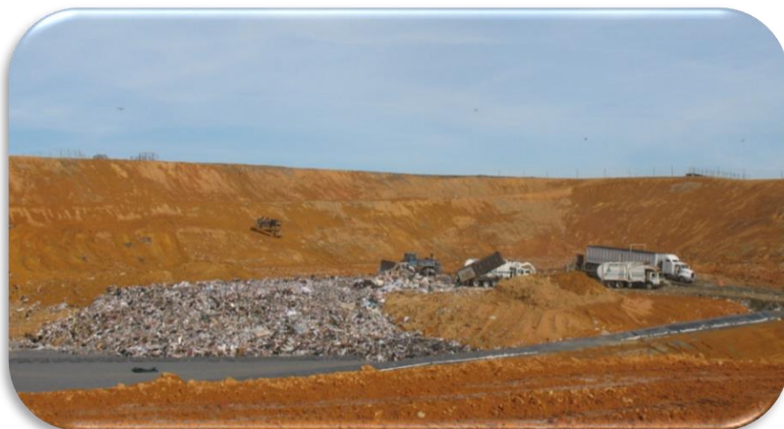
Mountain View Landfill face/dump area
